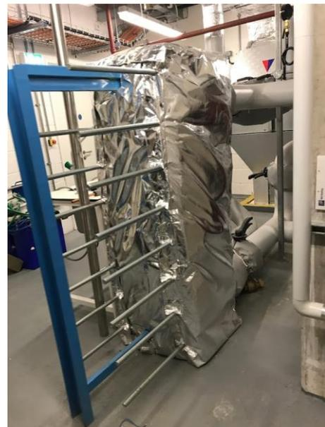
Figure 7.4b CHP LTHW Plate Heat Exchangers
