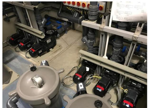
**Figure 6.5.1b Typical Water Circulation Pumps – Zone 1**
