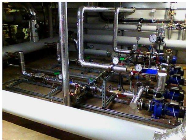
Figure 7.2a North Building Plant Room Thermal Insulation
