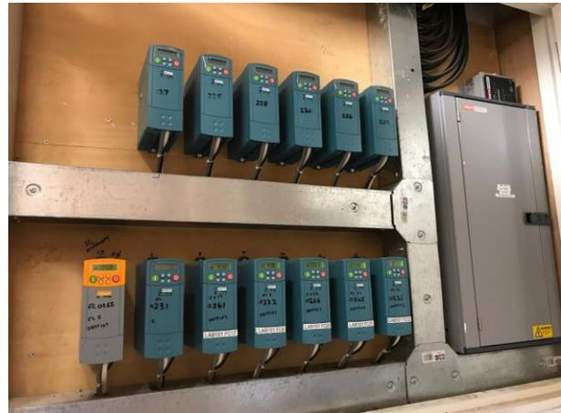
Figure 6.1.4d Lab 101 Fume Cupboard VSD Controls
