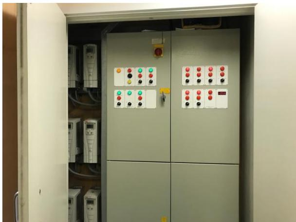
Figure 6.1.4a Lab 101 AHU Control Panel
